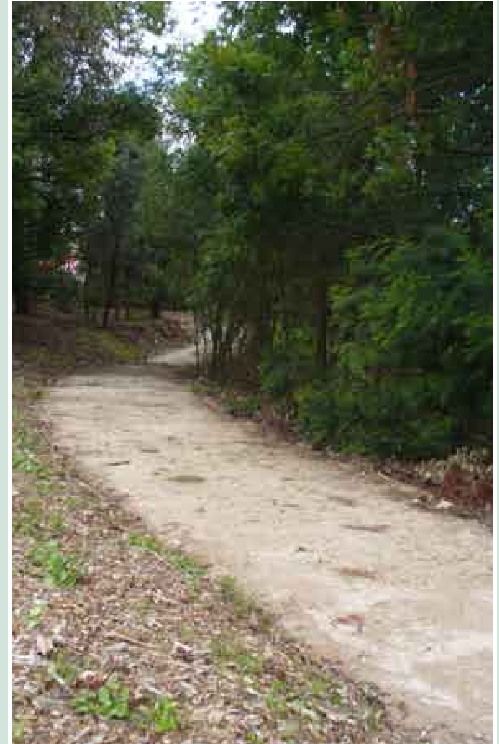
Newly completed section of the Redbank Track
